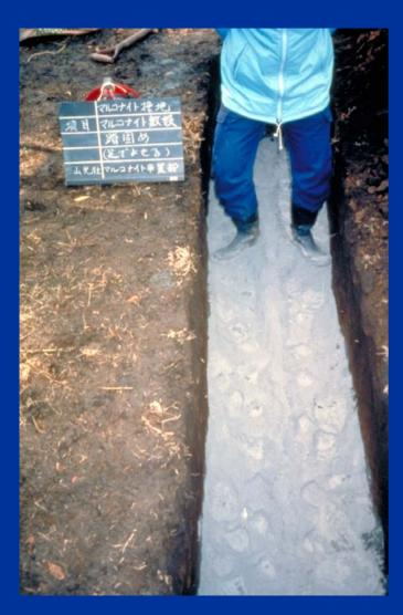
Lift the wire slightly to allow the SAN-EARTH to get under it encircling the conductor.
